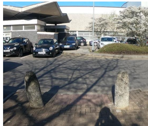
Pedestrian crossing and dropped curb missing at adjacent crossing point.
