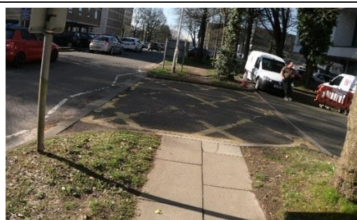
Pedestrian path ends without a crossing or onward path.
