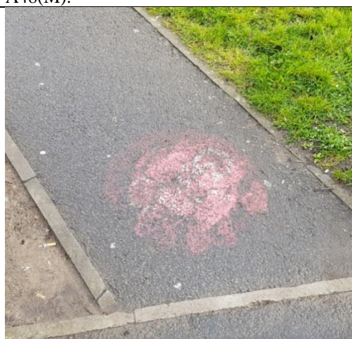
Cycle road markings badly worn making purpose unclear.
