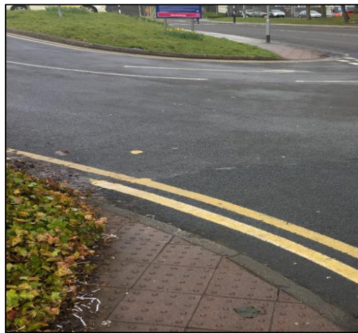
Long pedestrian crossing with incorrect tactile paving used.
