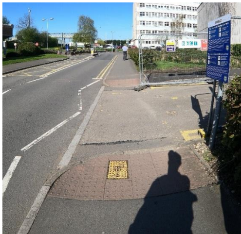
Incorrect tactile paving used outside Emergency Unit – indicating that this is a controlled crossing.
