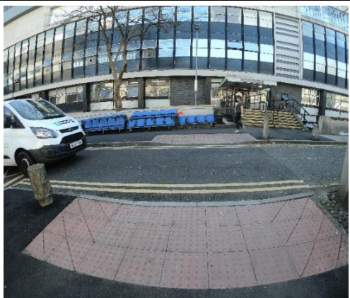
Incorrect tactile paving colour used at staff entrance off Academic Avenue.
