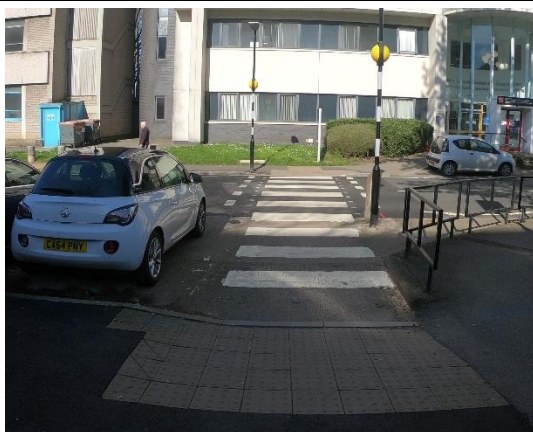
Incorrect colour tactile paving used on Academic Avenue outside Heart Research institute.
