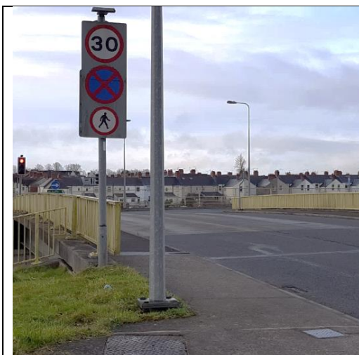
Unclear pedestrian signage on bridge over A48(M).
