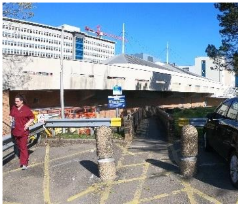
Narrow pedestrian/wheelchair access to main hospital building, not wide enough for two wheelchairs to pass.
