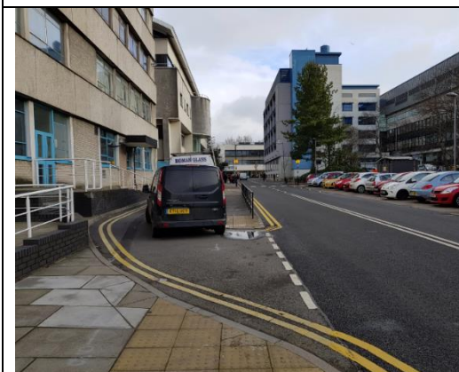
Narrow vehicle drop off bay causing vehicle to overlap onto footway.
