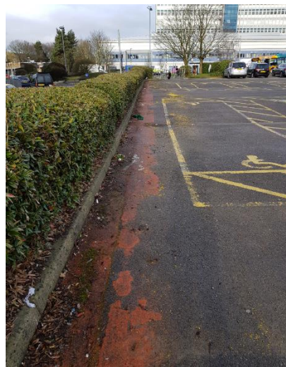
Poorly marked and narrow pedestrian path.
