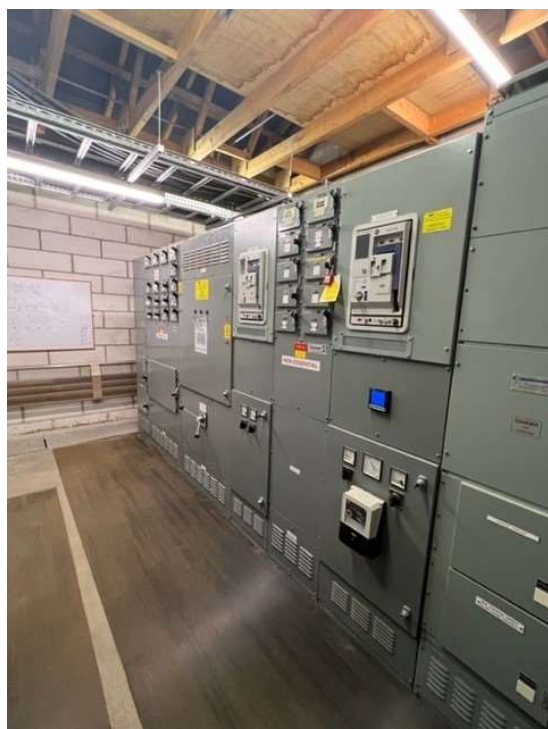
Figure 59: LV 20 Switchboard, now obsolete & not WHTM06-01 compliant
