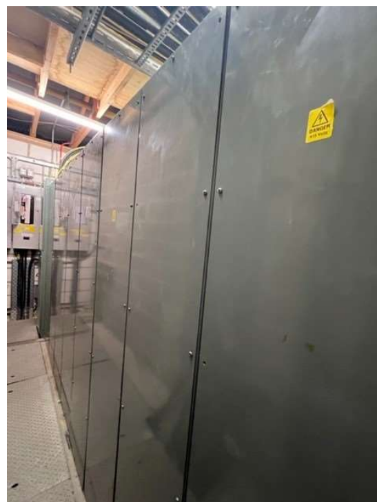
Figure 60: Warning labels installed rear of switchboard.
