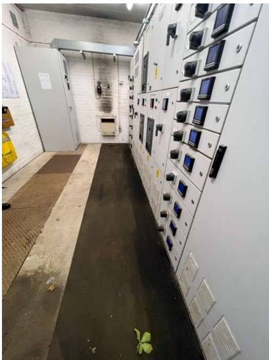
Figure 41: No rubber insulated mat installed in front of PFC Unit
