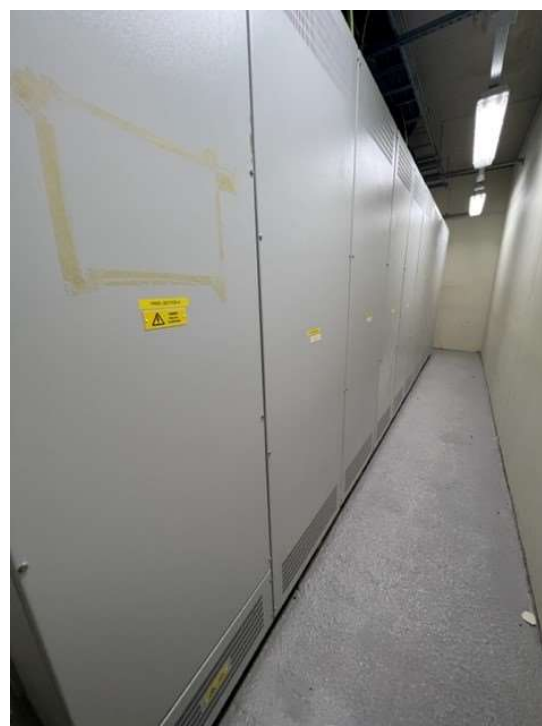
Figure 52: Warning labels installed rear of switchboard.
