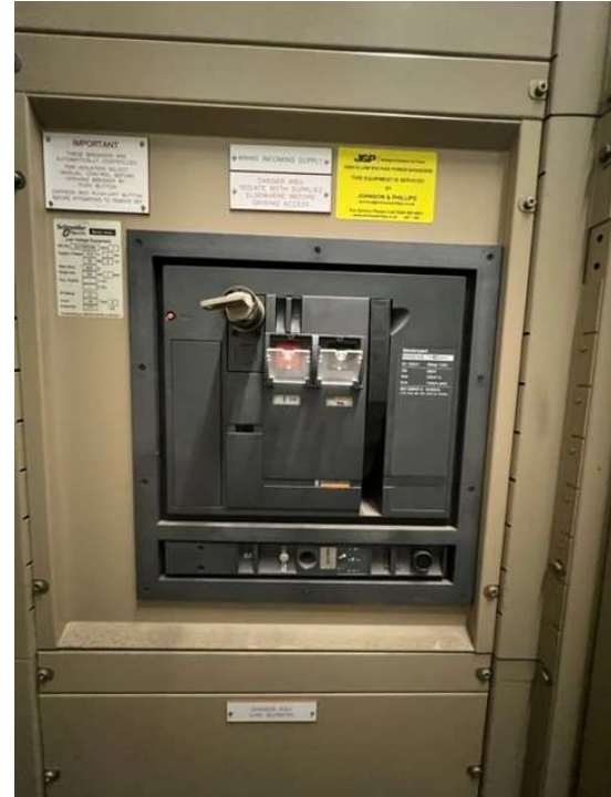
Figure 34: ACB no service label attached to identify if unit has been serviced.
