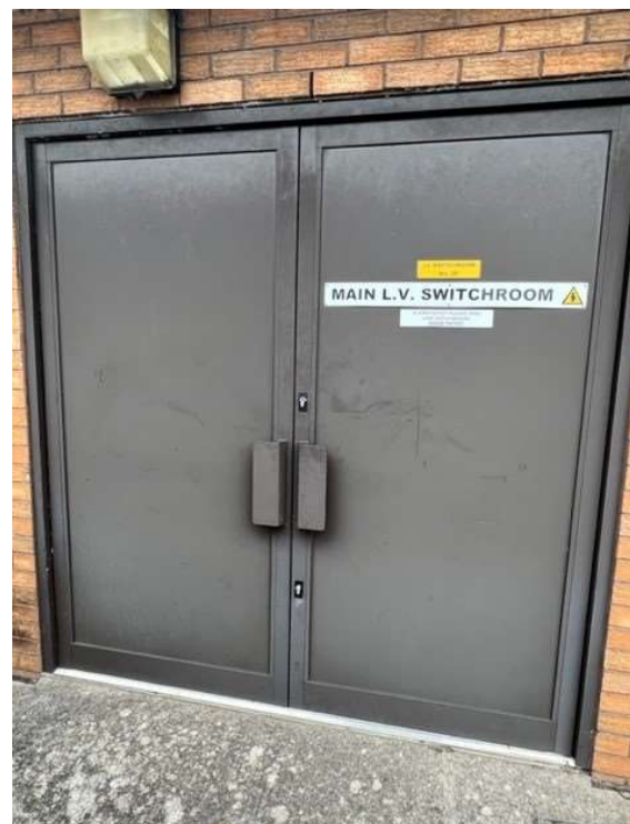
Figure 58: Entrance signage not fully HTM compliant
