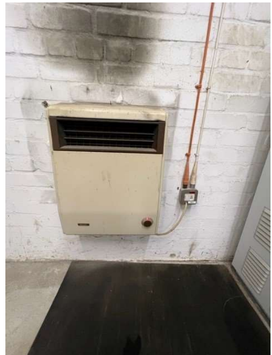
Figure 46: Electric heater (thermostatically controlled), signs of scorching
