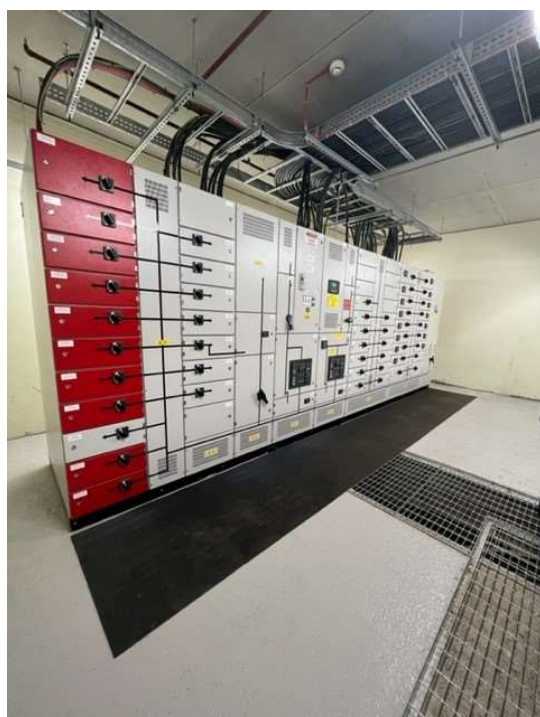
Figure 51: LV E Switchboard, not fully WHTM06-01 compliant.
