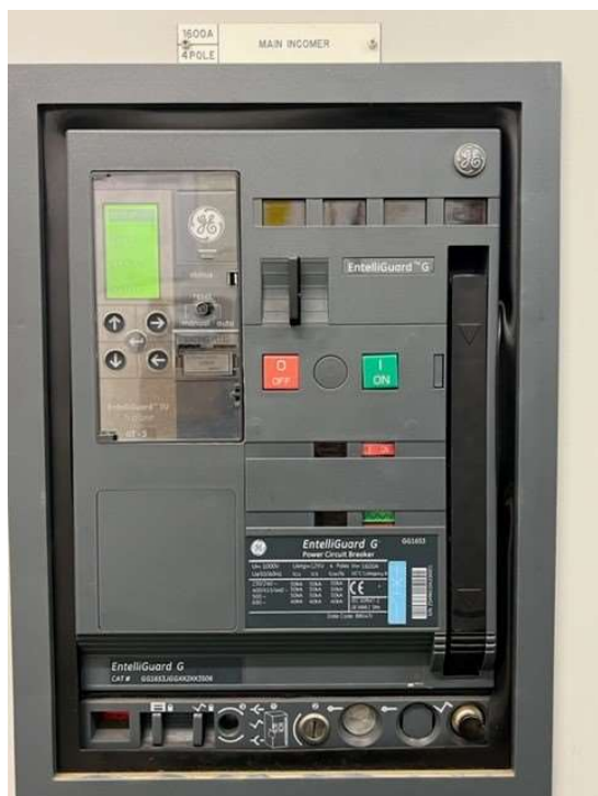
Figure 43: ACB no service label attached to identify if unit has been serviced.
