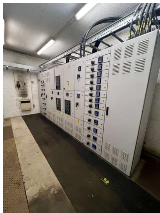
Figure 40: LV 5 Switchboard, not fully WHTM06-01 compliant
