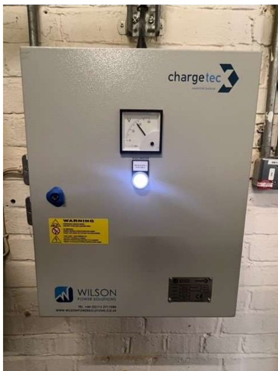
Figure 27: Tripping Battery, no service label attached
