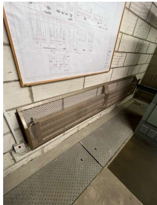
Figure 62: Electric Heater Installed & distribution Schematic on display
