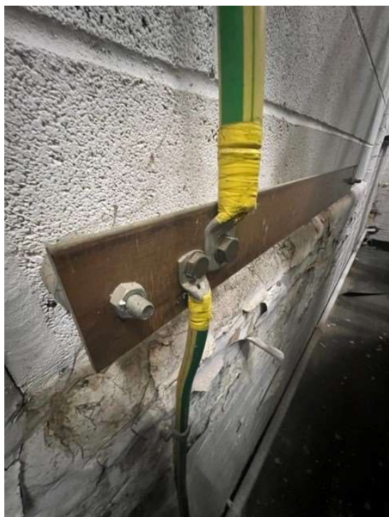
Figure 25: Earth Bar in good condition conductors unlabelled
