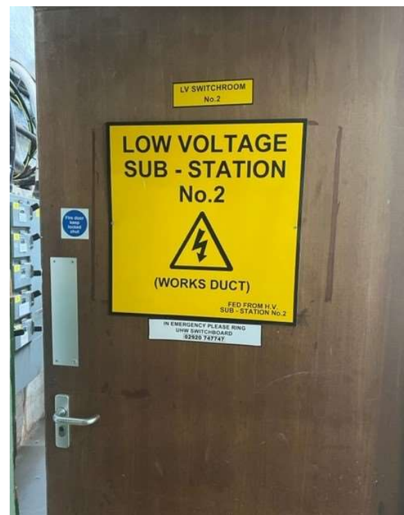
Figure 32: Entrance signage not fully HTM compliant
