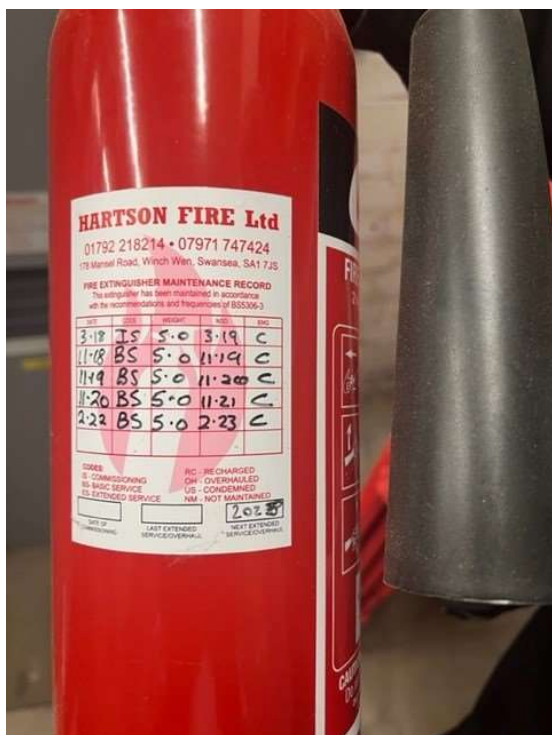
Figure 37: Co2 Fire Extinguisher date of last service February 2022
