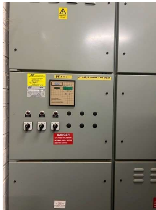
Figure 26: Power Factor Correction Unit switched off
