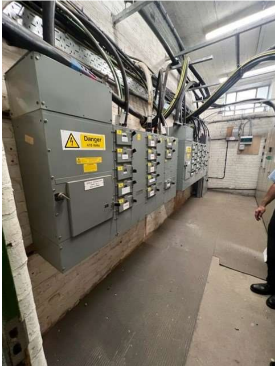
Figure 33: LV 2 Switchboard, now obsolete & not WHTM06-01 compliant
