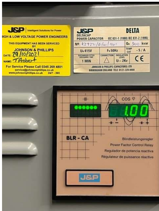
Figure 61: Powerfactor Correction Unit, service label dated 29/10/2021
