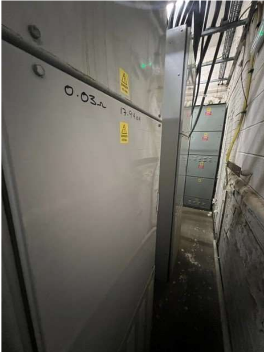
Figure 21: Warning labels installed rear of switchboard
